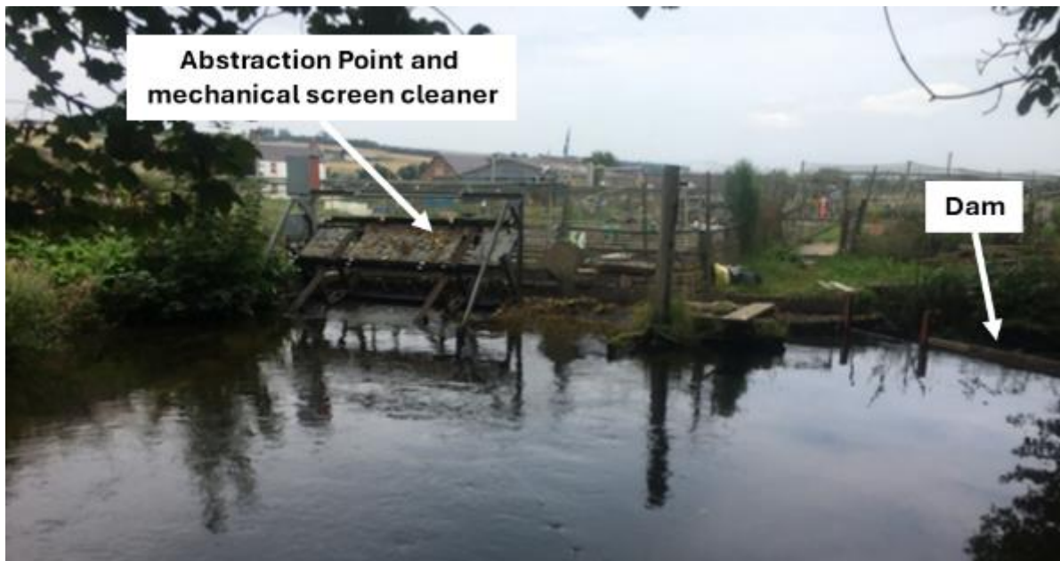
Figure 3 – West Mill Fish Farm abstraction point, mechanical screen cleaner and dam
