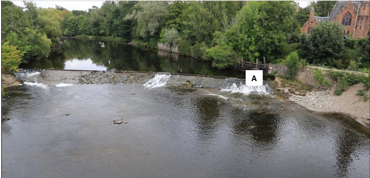
Figure 9 – At low river levels , flow over the weir diminishes markedly. A by-wash will be necessary close to the gates and proposed smolt screens (Point A) to allow smolts an escape route
