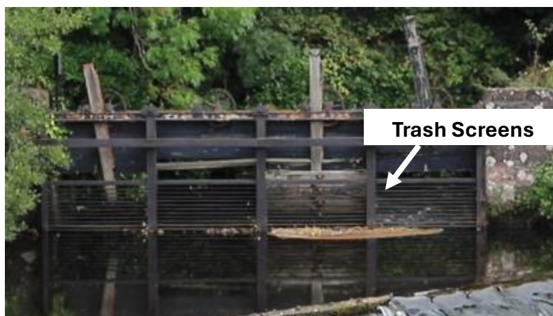
Figure 8 - A close up of the gates showing the trash screens. These stop heavy logs crashing into the gates during spates and also act as screens to stop adult fish entering the lade
