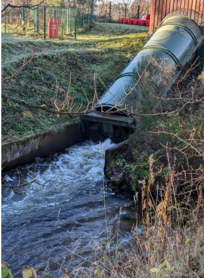
Figure 2 – The Hydro turbine – an Archimedes screw system which allows smolts to enter and journey through the screw
